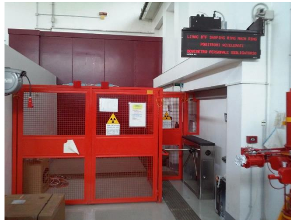
Fig. 13 - Example of access control equipment in DAΦNE, LNF, Italy.
